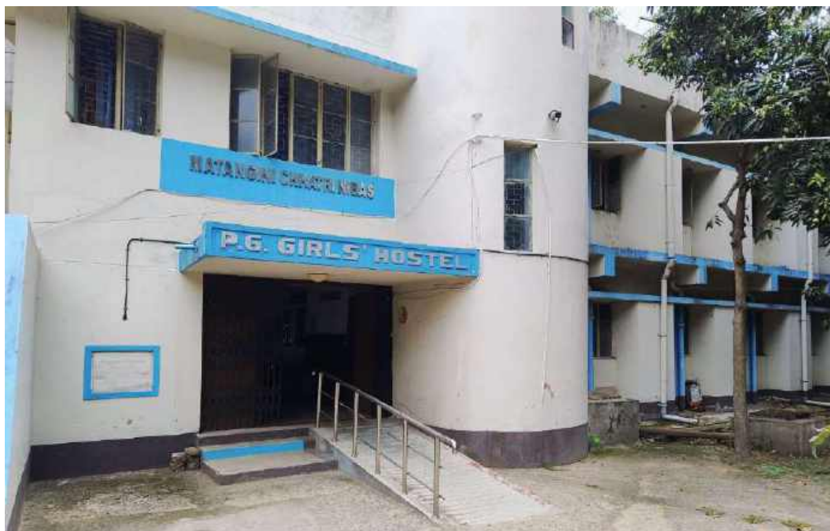
Figure 4: CCTV Camera installed at the Entrance of Girl's Hostel in the Vidyasagar University campus
